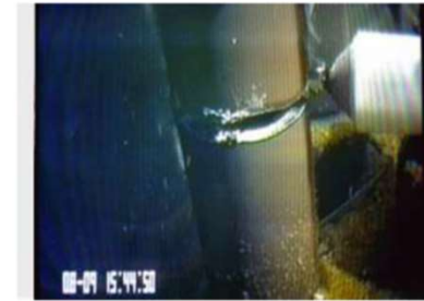
Plasma Arc Cutting of Control Rod Guide Tube
